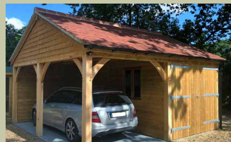
2 Bay Carriage House with oak on 2 elevations
