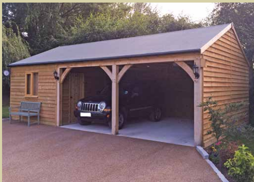
2 bay Carriage House with attached Workshop. 22° felt roof.
