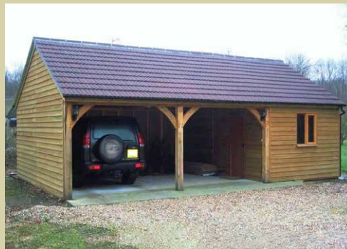
2 bay Carriage House with attached Workshop. 30° interlocking concrete tile roof.
