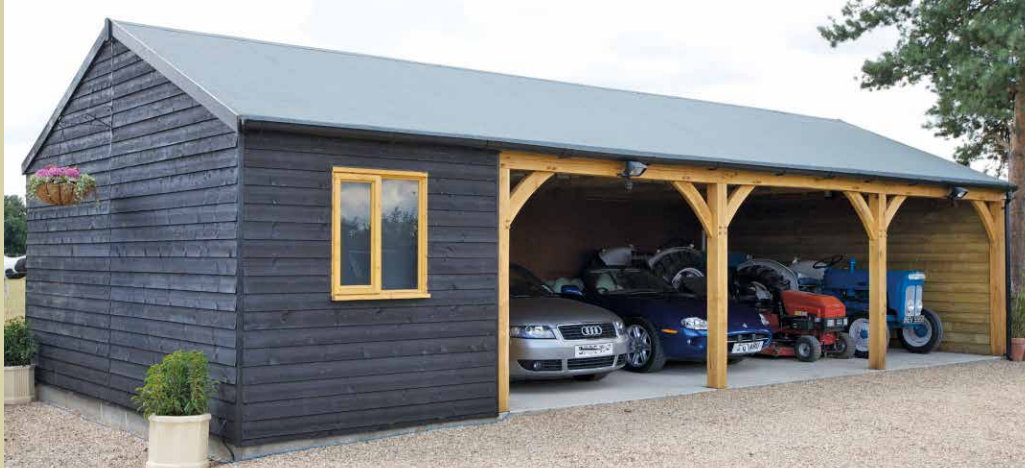
3 bay Carriage House with attached Workshop. 22° felt roof.
