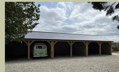
6 Bay Carriage House
