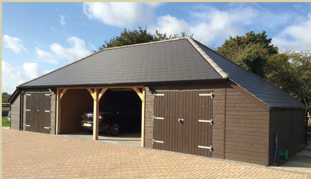
2 bay Carriage House with attached Cart Lodge at both ends. 35° fibre cement slate roof.
