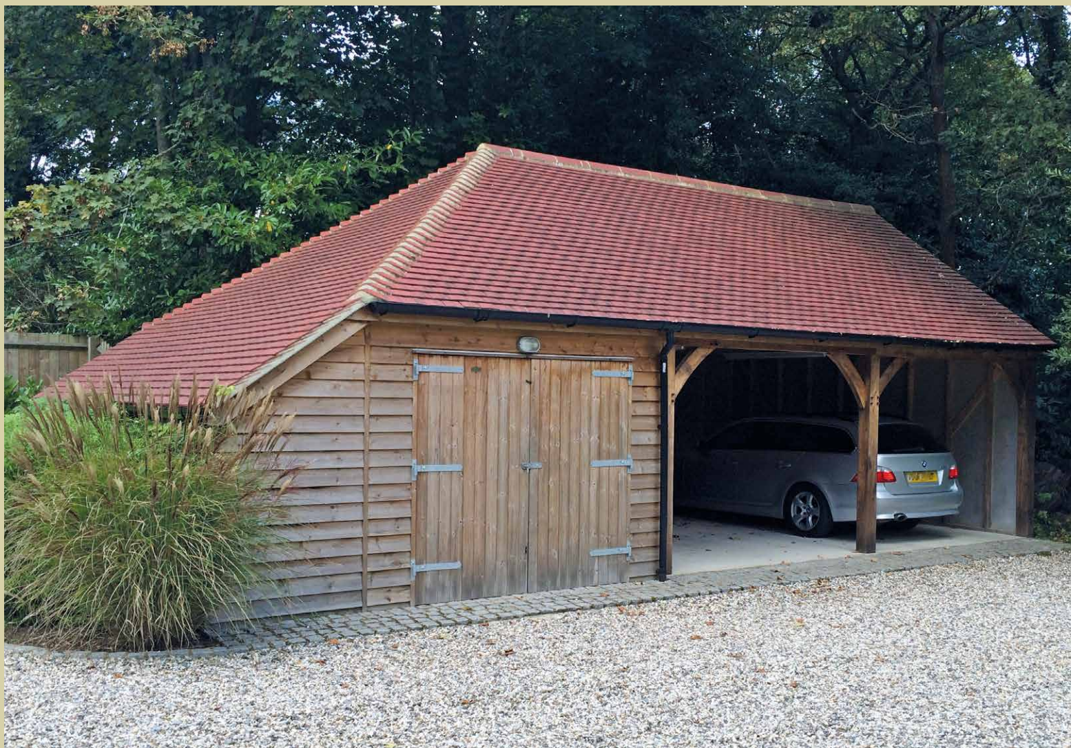
2 bay Carriage House with attached Cart Lodge. 35° plain tile roof.
