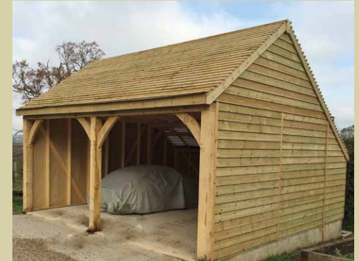
5.4 x 5.4 two bay Open Barn. 35° Batted and felted, awaiting tiles.
