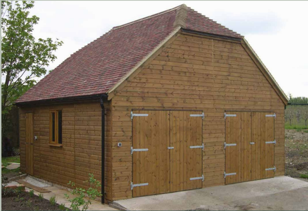
Double Garage. 35° plain tile roof and optional barn hips, personal door and window.
