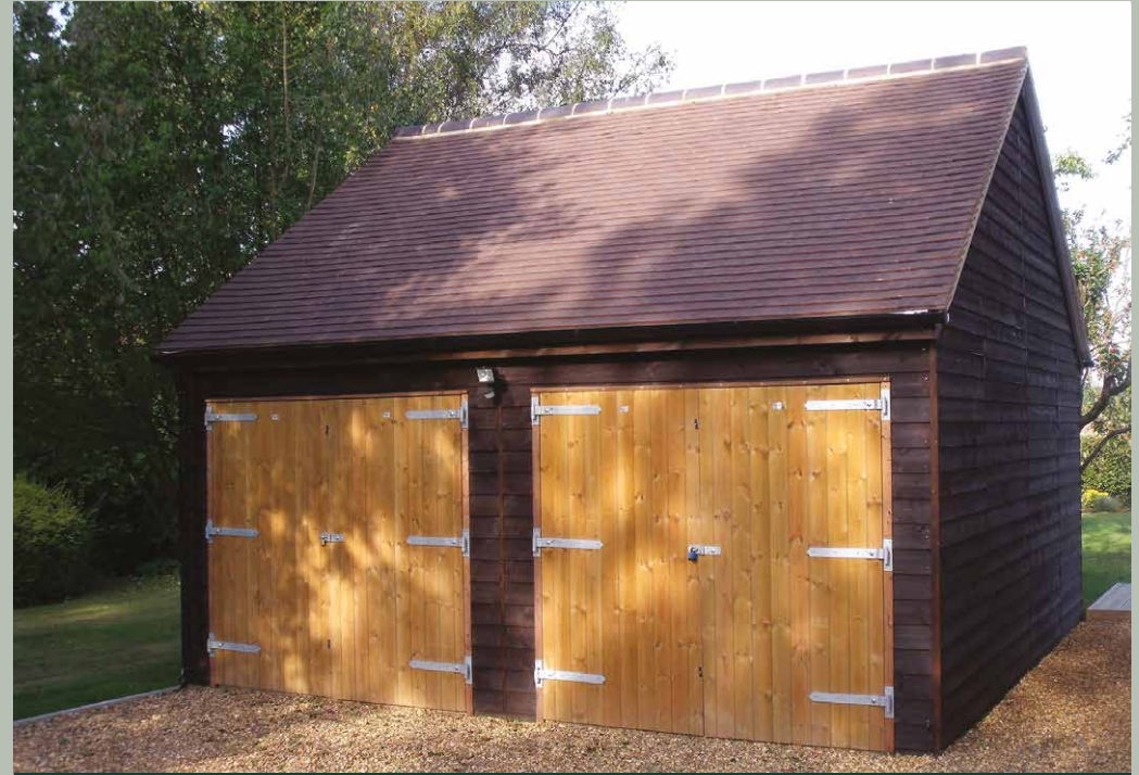
Double Garage. 35° plain tile roof. 2.4m eaves height (doors in side elevation).
