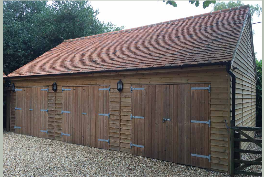
Triple Garage. 35° plain tile roof. 2.4m eaves height (doors in side elevation).
