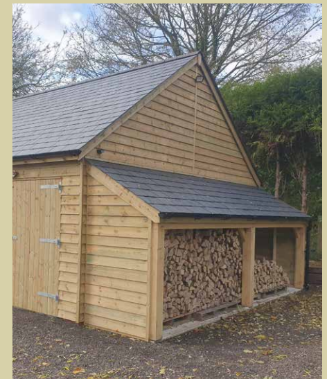
Log Store with natural slate roof.
