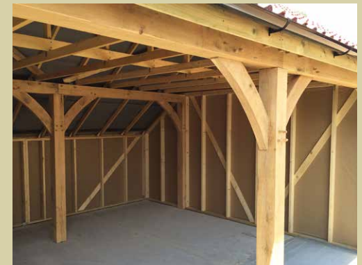
Inside view of Open Barn.
